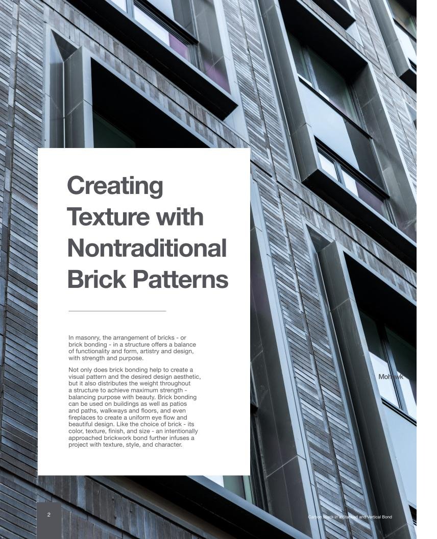
Although there is a wide variety of patterns, let's explore the six most popular types of brick bonds commonly used for walls. These bonds each use a stretcher brick - a brick laid flat, exposing its longer, narrow side – and/or header bricks - a brick laid flat with the shorter, squared face exposed.
